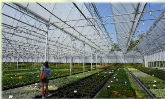
Figure 12: Glasshouse: roof and sides open completely to provide protection from the elements
